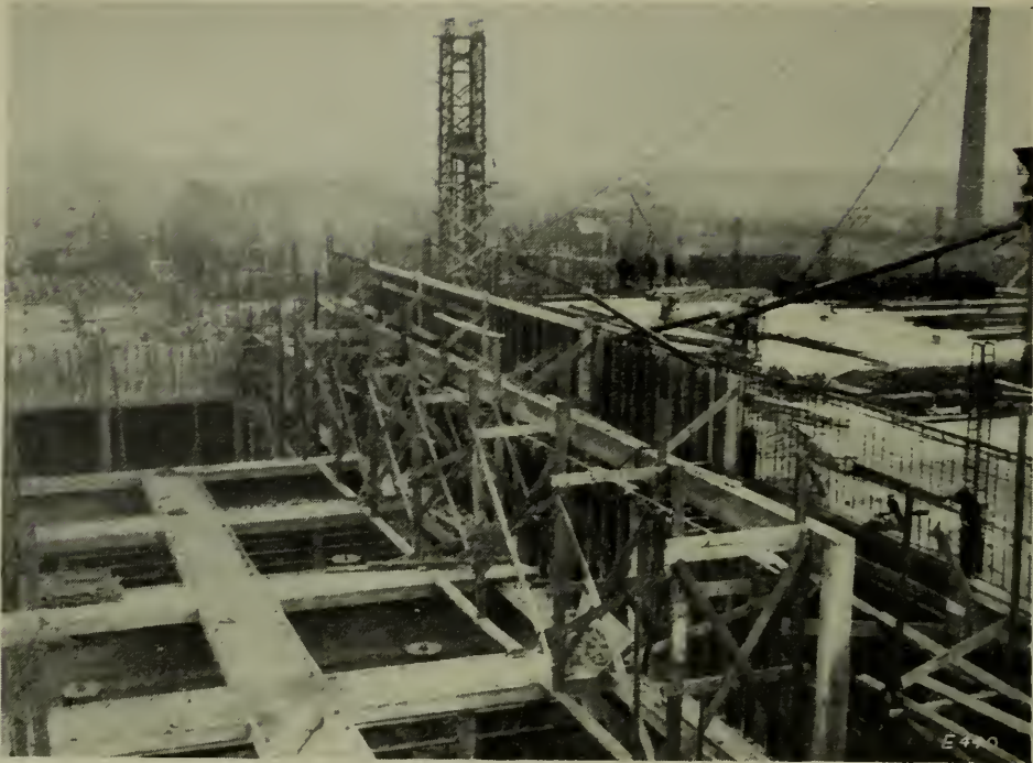
CATCH BOXES AND ADJACENT PURIFIER HOUSE UNDER CONSTRUCTION.
